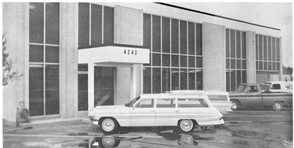
Houston branch of Southwest Sales Division (formerly Earl Lipscomb Associates) has just moved into ground floor of this new building.
